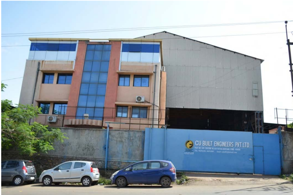
Head Office and Manufacturing Unit 1 (Machining Facility)
