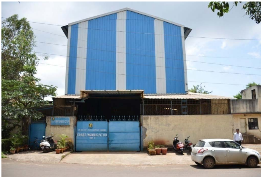
Unit 2 (Assembly Unit)
